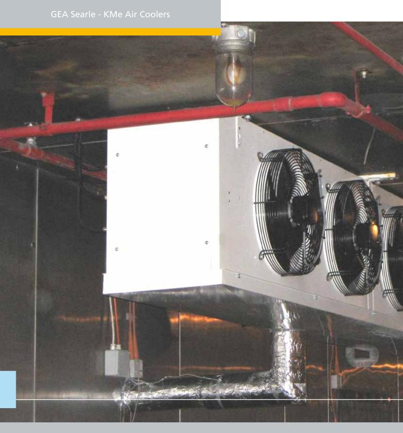
The KMe range of coolers is ideally suited to largecold rooms and small ware-houses where an efficient solution is required. The KMe can also be used for industrial food processing and agricultural applications.
